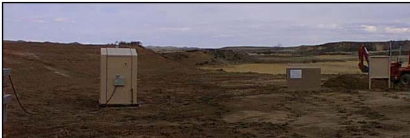
*Natural Gas Wellhead – tall enclosure houses microturbine*
