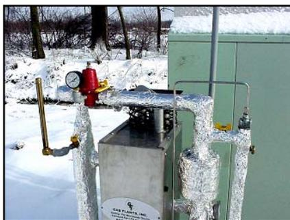
*Vaporiser with pipe insulation*
